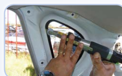
Access confined spaces
